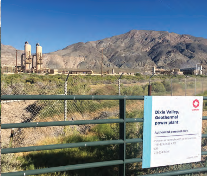
Construction of a geothermal plant in Dixie Valley has halted over concerns for the endangered Dixie Valley toad.
